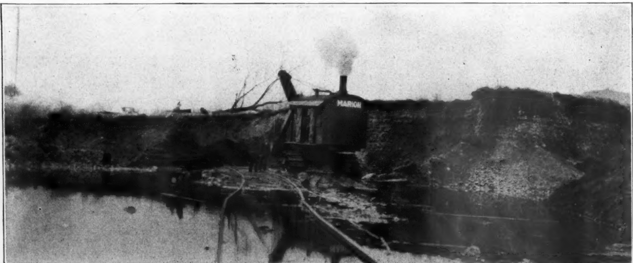
Excavating the Bank at the Second Operation with a Steam Shovel.
